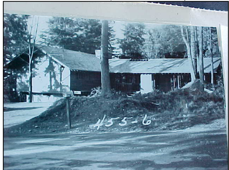
Figure 5 • Northwest Contemporary House (1953) designed by architect Dan F. Miller.
